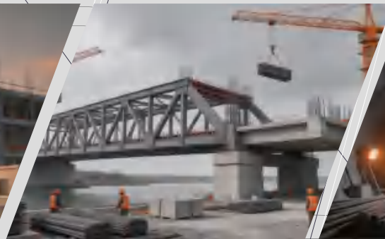
桥梁建设 Bridge Construction
