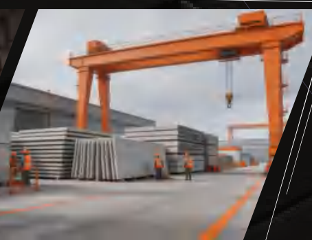
预制构件厂 Precast Component Factory
