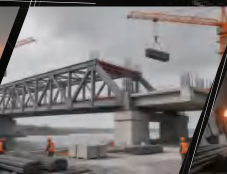
桥梁建设 Bridge Construction
